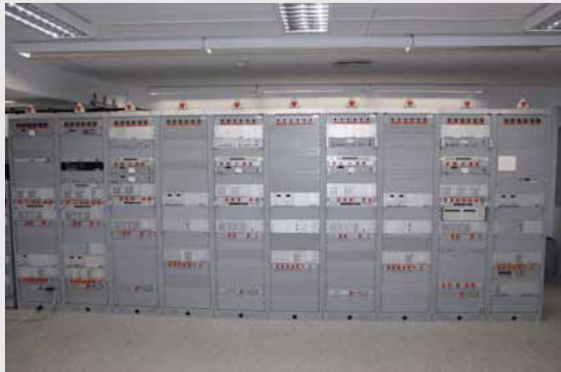
Part of radio transmission station
