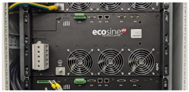
Figure 13-1 Example of a power module with all cables and fixation screws removed
